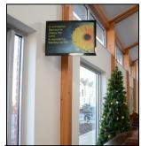
27" Asus relay LCD mounted on a side wall Z-bracket - allowing musicians to view song words and images from the platform.
